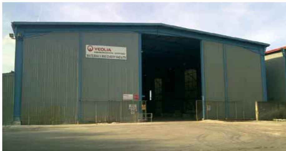
Veolia Materials Recovery Facility (MRF) in Port Kembla
