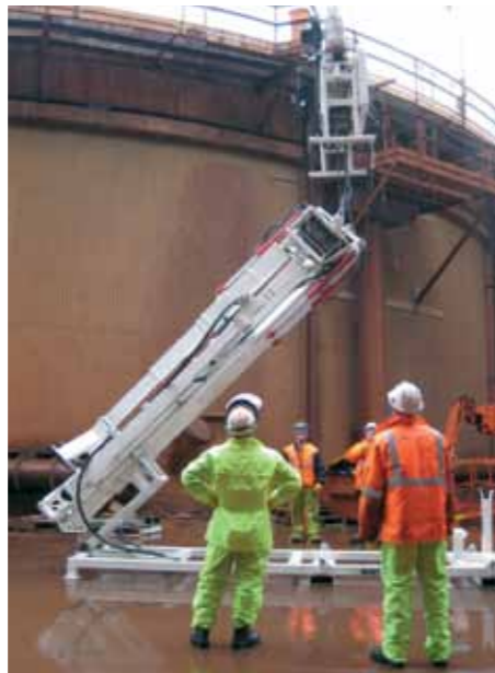
R125 Descale Rig being lifted from the transport cradle
