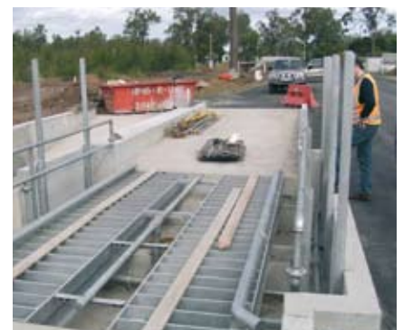
Construction of the New Cell
